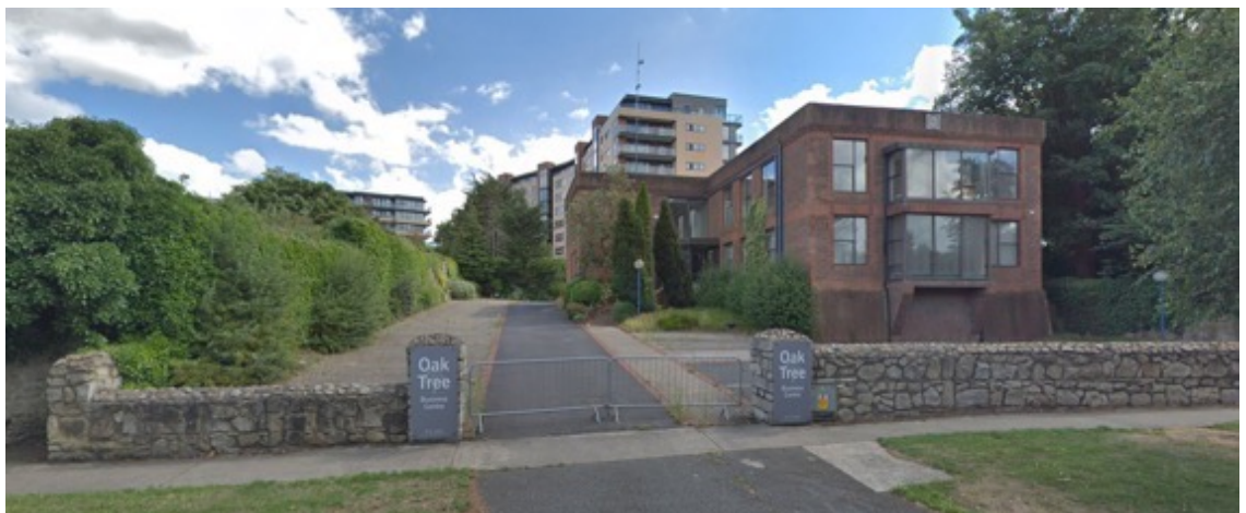
Figure 12 - View of Oaktree Business Centre - to be demolished
